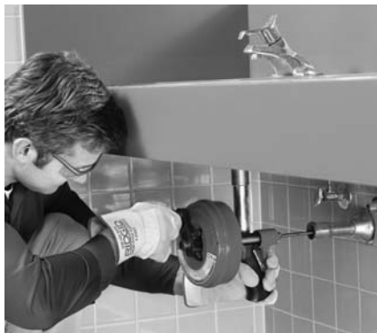
Figure 8 – Power-Spin Used By Hand
